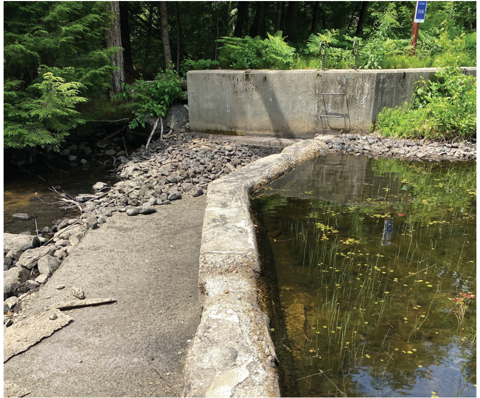
Above: Winter damage to the top of the dam. At right: Stumps of newly-cleared pines are visible above the abutment. / Pen Hallowell
